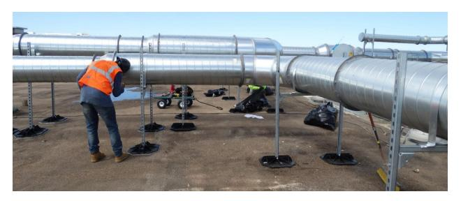
It's Durable! Sheet metal ducts, and particularly spiral ducts, are proven to be durable in outdoor applications. Other rooftop products have been introduced, including some made with phenolic board. Most are simply one or two layers of insulating board with an external lagging applied. These have neither the strength nor durability of
