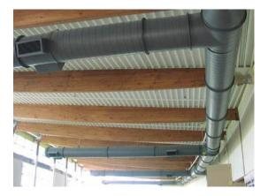
SPOT Flanges<sup>™</sup> are an economical option for joining round and flat oval spiral pipe and fittings where the size or an installer preference requires a flanged connection. They are roll-formed from 18-gauge galvanized material, then factory mounted on our spiral pipe and fittings by spotwelding and sealing. Field connections are made using neoprene gaskets or butyl tape (by others) placed between flanges, then screwed together on 6-inch centers.
